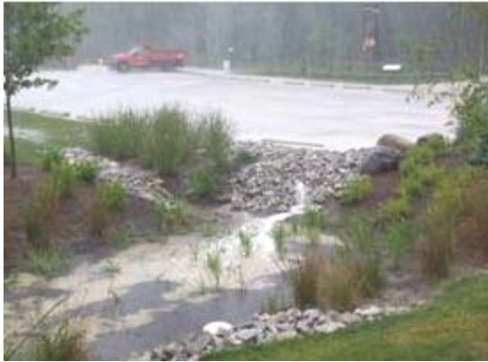
Rain Gardens capture runoff and Recharge Groundwater.
